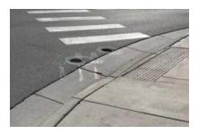
Potholes – created as a safety procedure during the locate work to visibly confirm where utilities lines are underground. The holes are backfilled temporarily until a permanent patch is made, usually within 24 hours.
