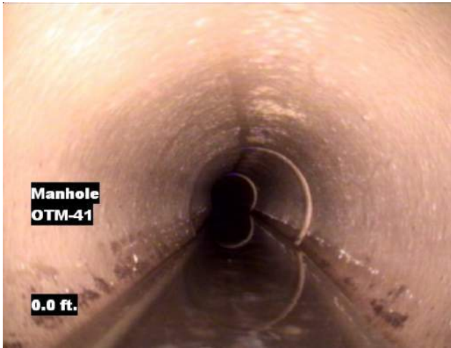
Manhole OTM-41 0.0 ft. Distance: 0.0 ft. Grade: 0 Condition: Manhole Remarks: OTM-41
