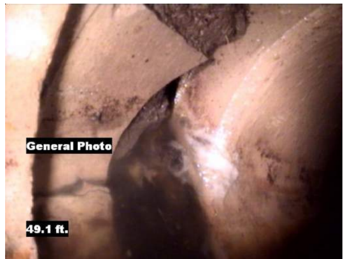
General Photo 49.1 ft. Distance: 49.1 ft. Grade: 0 Condition: General Photo Remarks: N/A
