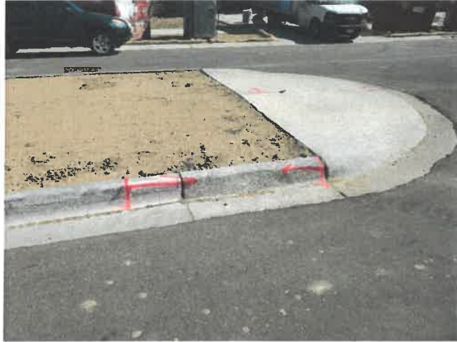
Image 16 – Chipped curb – Remove/replace curb and gutter to nearest control joint.
