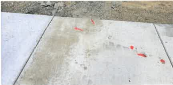
Image 33 (2639) – Fly Ash and other Debris imbedded in ramp – Clean up
