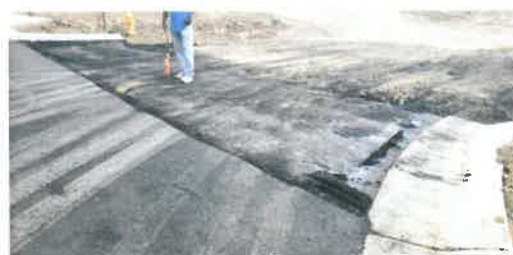
Image 37 (3917) – Top lift of asphalt not completed to end of curb return – Complete with next phase. Revised July 27, 2020
