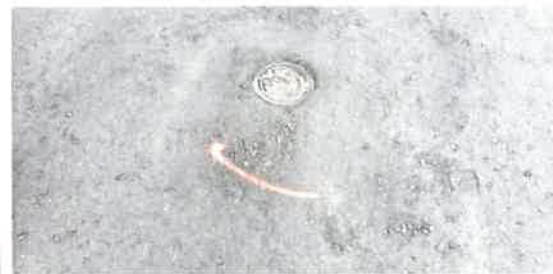
Image 38 (4105) – Poorly patched asphalt around valve box – Mill and overlay, monitor during warranty period.
