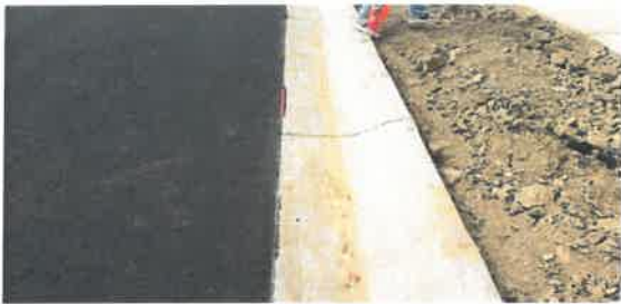
Image 29 (2347) – Chipped curb – Monitor during warranty period. Revised July 27, 2020
