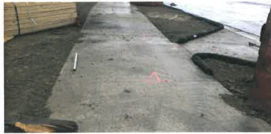
Image 48 (5402) – Ponding of storm drainage in ramp - Remove/replace walk and curb ramp
