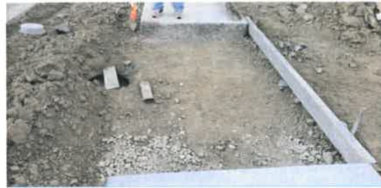
Image 22 (1407) – Missing sidewalk – Install.
