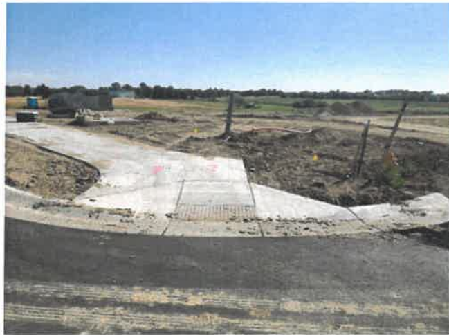
Image 8 – ADA Ramp on northeast corner of Park Street and Lake Helen is not complete, and the sidewalk above the ramp is not ADA Compliant – Remove/replace.
