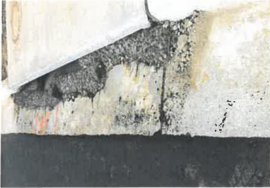
Image 27 (2239) – Asphalt on top of curb and gutter – Clean up.
