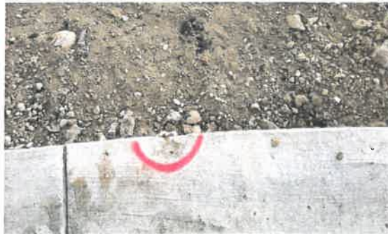
Image 44 (4631) – Chipped in curb and gutter – Monitor during warranty period. Revised July 27, 2020
