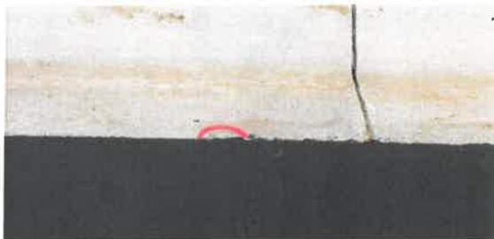
Image 29 (2347) – Chipped curb – Monitor during warranty period. Revised July 27, 2020
