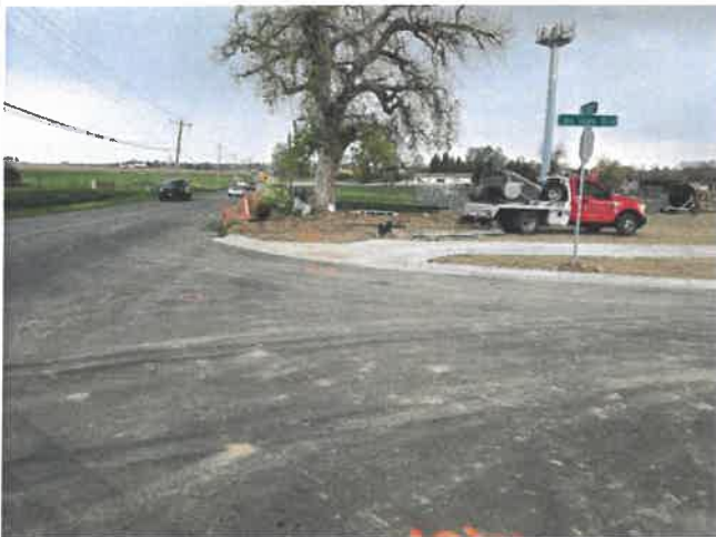
Image 7- Developer did not install culvert and roadside ditch on north and south side of Lake Helen to fix steep drop off from 3 rd Street to the Ditch, as discussed.
