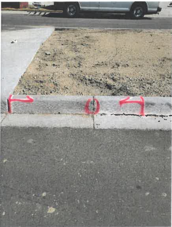
Image 15 – Crack/chip at control joint. Remove/replace curb and gutter to nearest joint.
