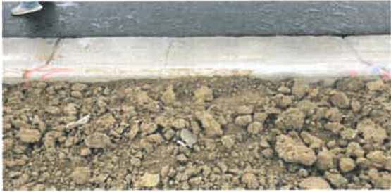
Image 47 (5311) – Pitted concrete sidewalk from pour during rain – Remove/replace for final acceptance
