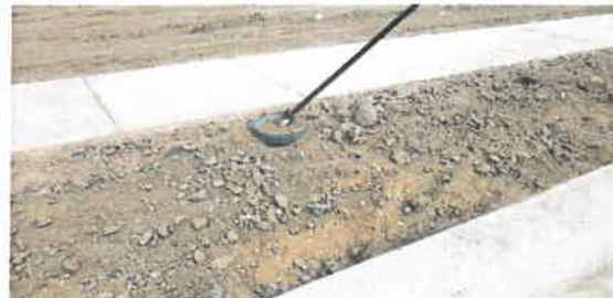
Image 30 (2425) – Meter pit box adjustment – Adjust to finished grade.
