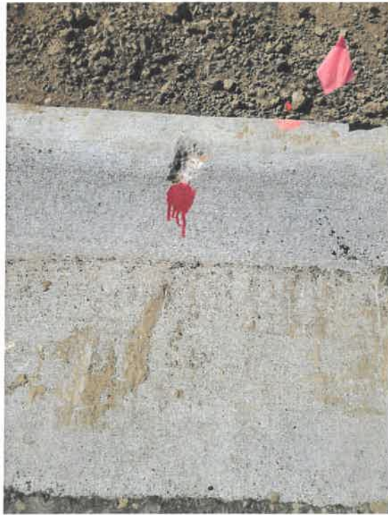
Image 16 – Chipped curb – Remove/replace curb and gutter to nearest control joint.
