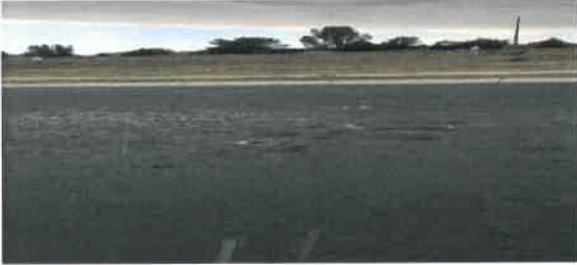
Image 19 (1034) – Chipped concrete – Remove/replace stone to nearest control joints.
