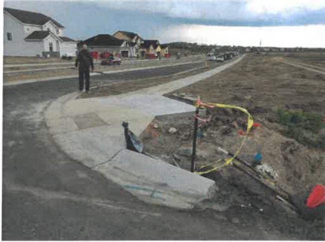
Image 8 – ADA Ramp on northeast corner of Park Street and Lake Helen is not complete, and the sidewalk above the ramp is not ADA Compliant – Remove/replace.
