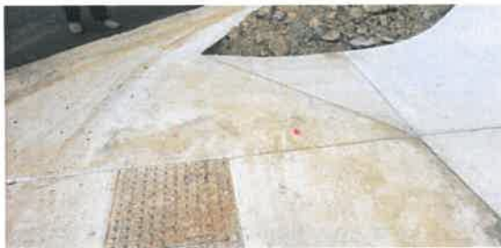
Image 35 (3601) – Chip in concrete walk – Monitor during warranty period. Revised July 27, 2020
