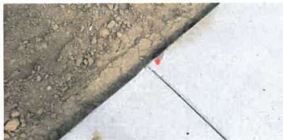
Image 37 (3917) – Top lift of asphalt not completed to end of curb return – Complete with next phase. Revised July 27, 2020
