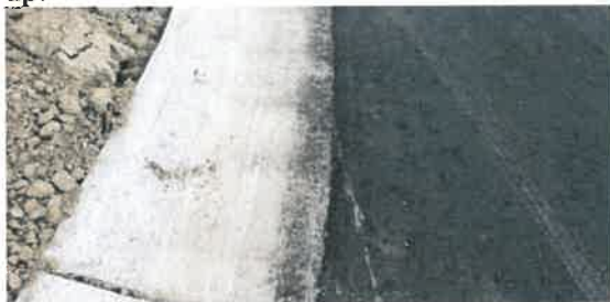
Image 21(1344) – Asphalt on curb and gutter-Clean up.
