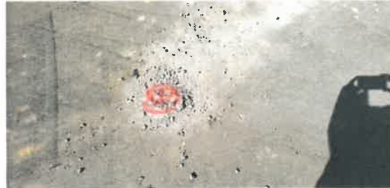
Image 20 (1129) – Hairline fracture in concrete – Monitor, remove/replace curb and gutter to the nearest control joints if fracture begins to increase in size.
