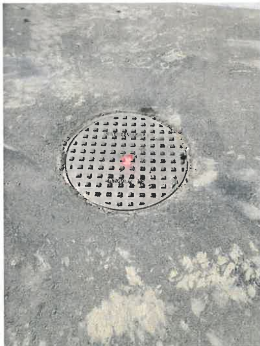
Image 11 – Wrong manhole lid – Replace with properly labeled lid.
