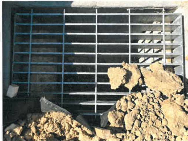
Image 12 – Poorly maintained erosion control on area inlet – Remove debris and properly set erosion control mechanism.
