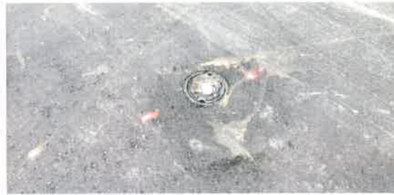
Image 36 (3818) – Fly Ash and other debris imbedded in ramp – Clean up.
