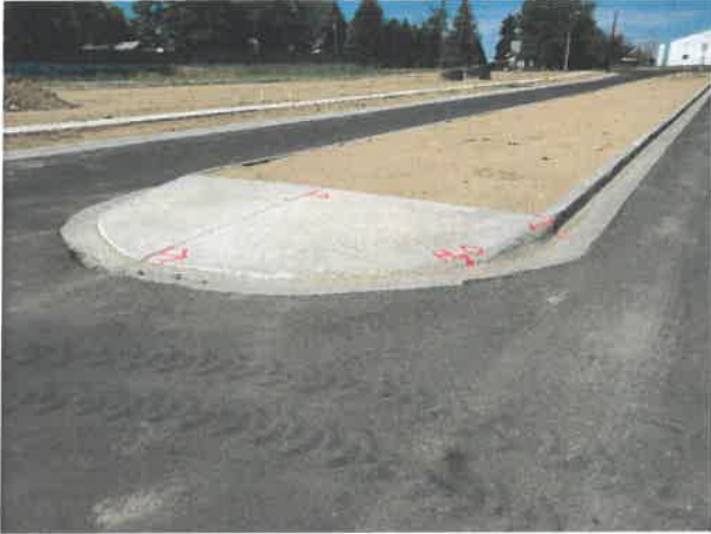
Image 15 – Crack/chip at control joint. Remove/replace curb and gutter to nearest joint.
