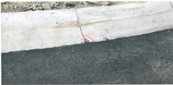
Image 21(1344) – Asphalt on curb and gutter-Clean up.
