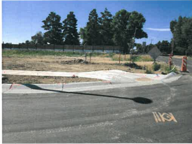
Image 12 – Poorly maintained erosion control on area inlet – Remove debris and properly set erosion control mechanism.
