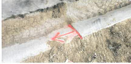
Image 48 (5402) – Ponding of storm drainage in ramp - Remove/replace walk and curb ramp
