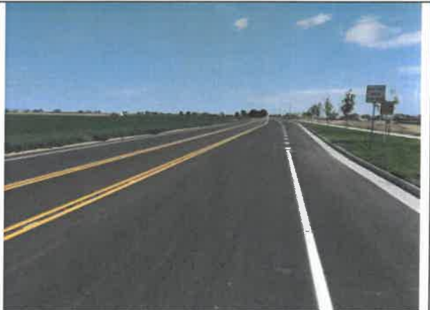
Image 6 – Lane widths along WCR 5 do not measure to be 12-foot wide. Striping widths do not measure to be 8-inches wide.
