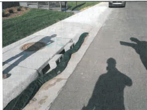
Image 1 – Damaged rock socks, typical in areas around site.
