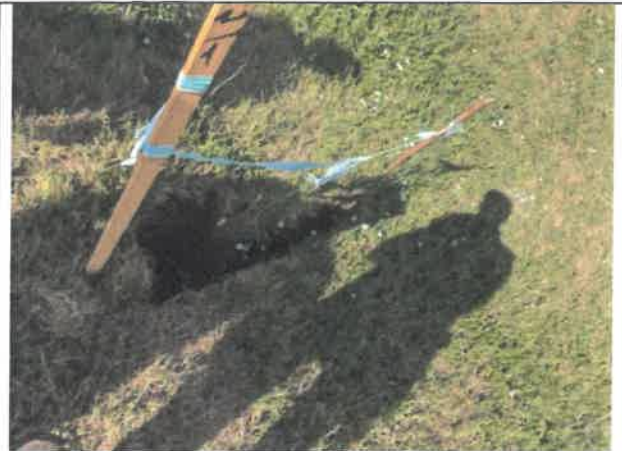
Image 4 – Open potholes along WCR 5 pose a trip / fall hazard
