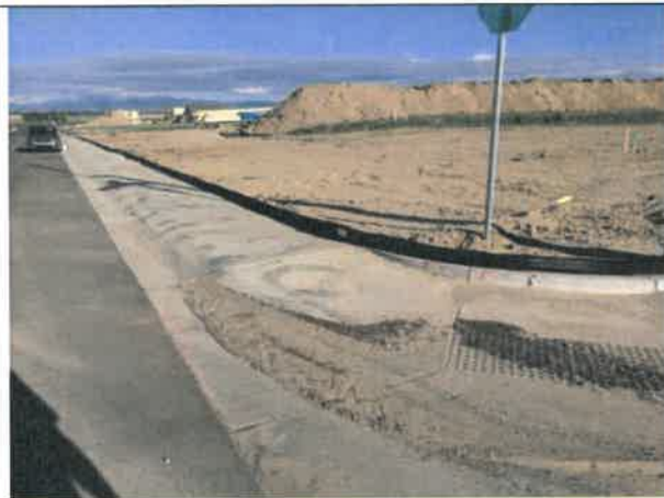
Image 1 – Low spot observed trapping sediment at northwest corner of Kerry Street and Longhorn Drive.
