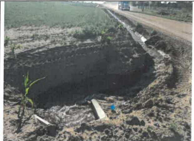
Image 4 – Unstabilized soils showing signs of erosion, riprap for FES missing at FES for irrigation ditch.
