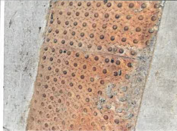
Concrete Clean up/seal all ADA ramps
