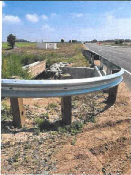
Guardrail needs to be secured and set
