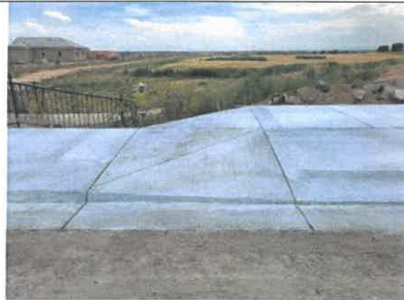
Concrete (Joint alignment)
