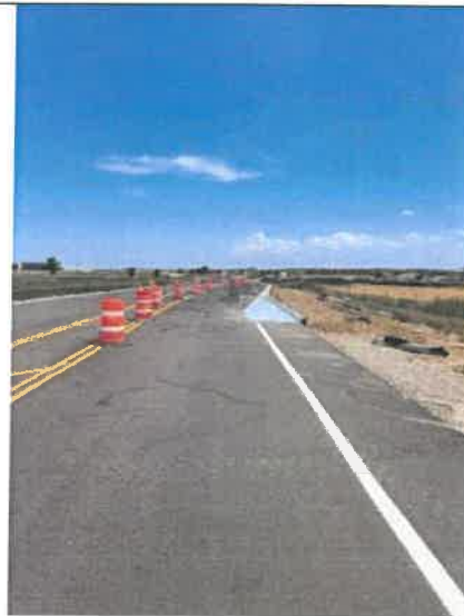
Concrete Item (No flaggers with traffic control)
