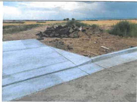
Concrete (Joint alignment) Backfill/Cleanup
