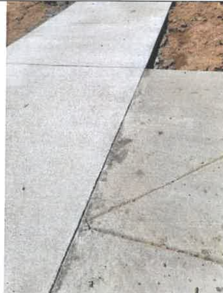
Concrete Clean up
