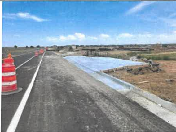
Concrete (Joint alignment)
