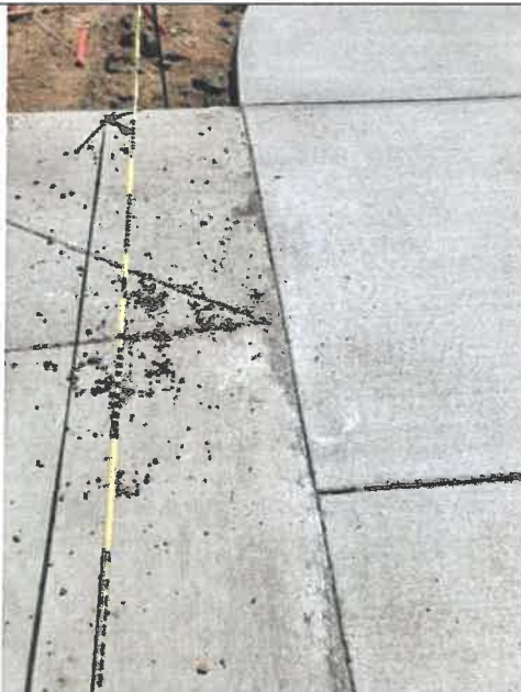
Concrete Clean Up
