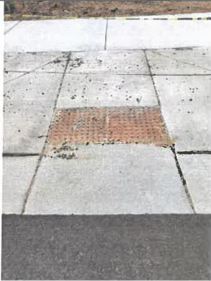
Concrete Clean up/seal all ADA ramps
