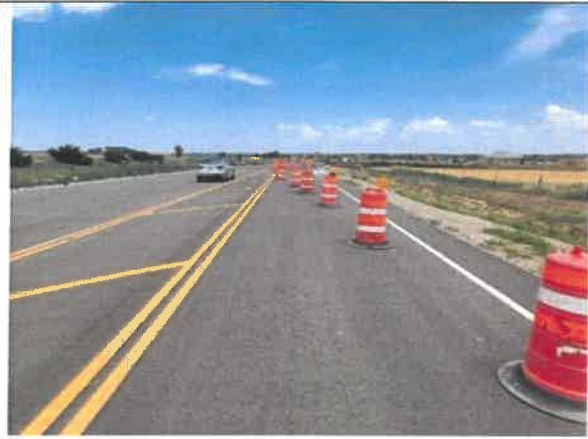
Concrete Item (No flaggers with traffic control)
