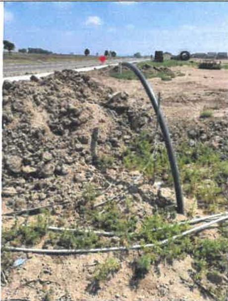
Utilities covered with peds Clean up
