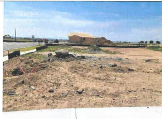
Utilities Exposed/Clean Up
