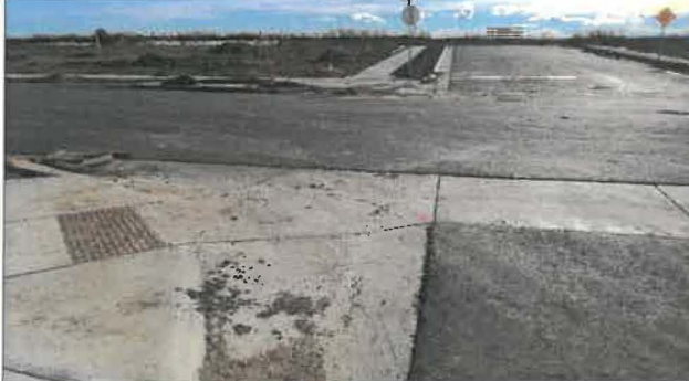
3- Seal Crack in cross pan on north side of intersection
