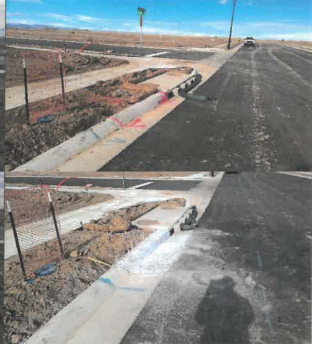
2- R&R @ inlet on west side of road south of Plum St
