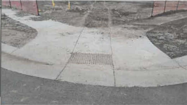
16- 2 cracks in ramp need to be sealed at Harvest Moon/Harvest Dr
