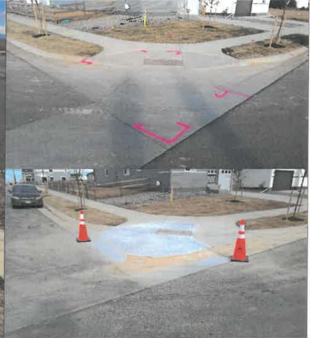
12- Ramp on NE corner of Red Barn Ave & Harvest Dr needs to be replaced
