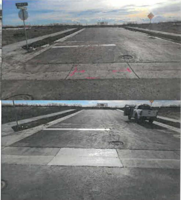
4- R&R cross pan on south side of intersection
