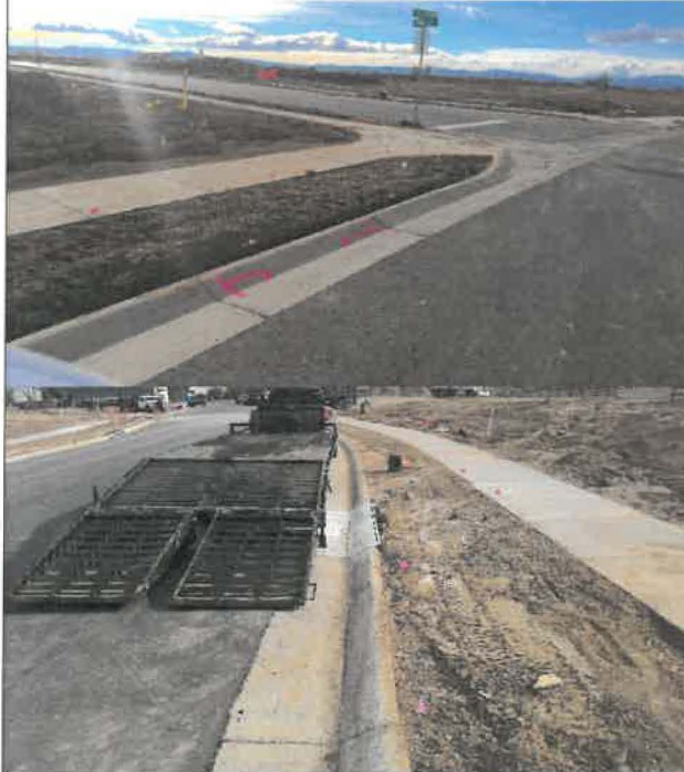
11- R&R c/g on Red Barn Ave (south side, east of intersection with Ranch St)
