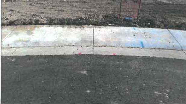
9- Seal crack at end of cul-de-sac
