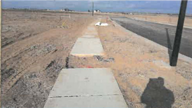
14- Sidewalk panel needs replaced- it was removed for street light install
