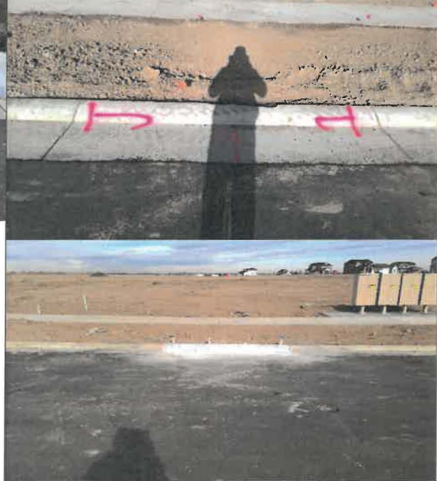
12- Ramp on NE corner of Red Barn Ave & Harvest Dr needs to be replaced
