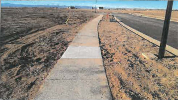
16- 2 cracks in ramp need to be sealed at Harvest Moon/Harvest Dr
