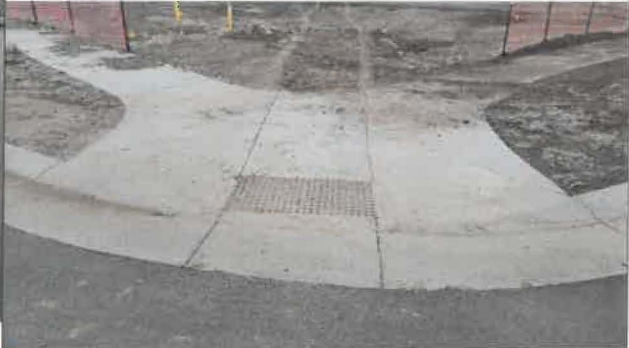
16- 2 cracks in ramp need to be sealed at Harvest Moon/Harvest Dr
